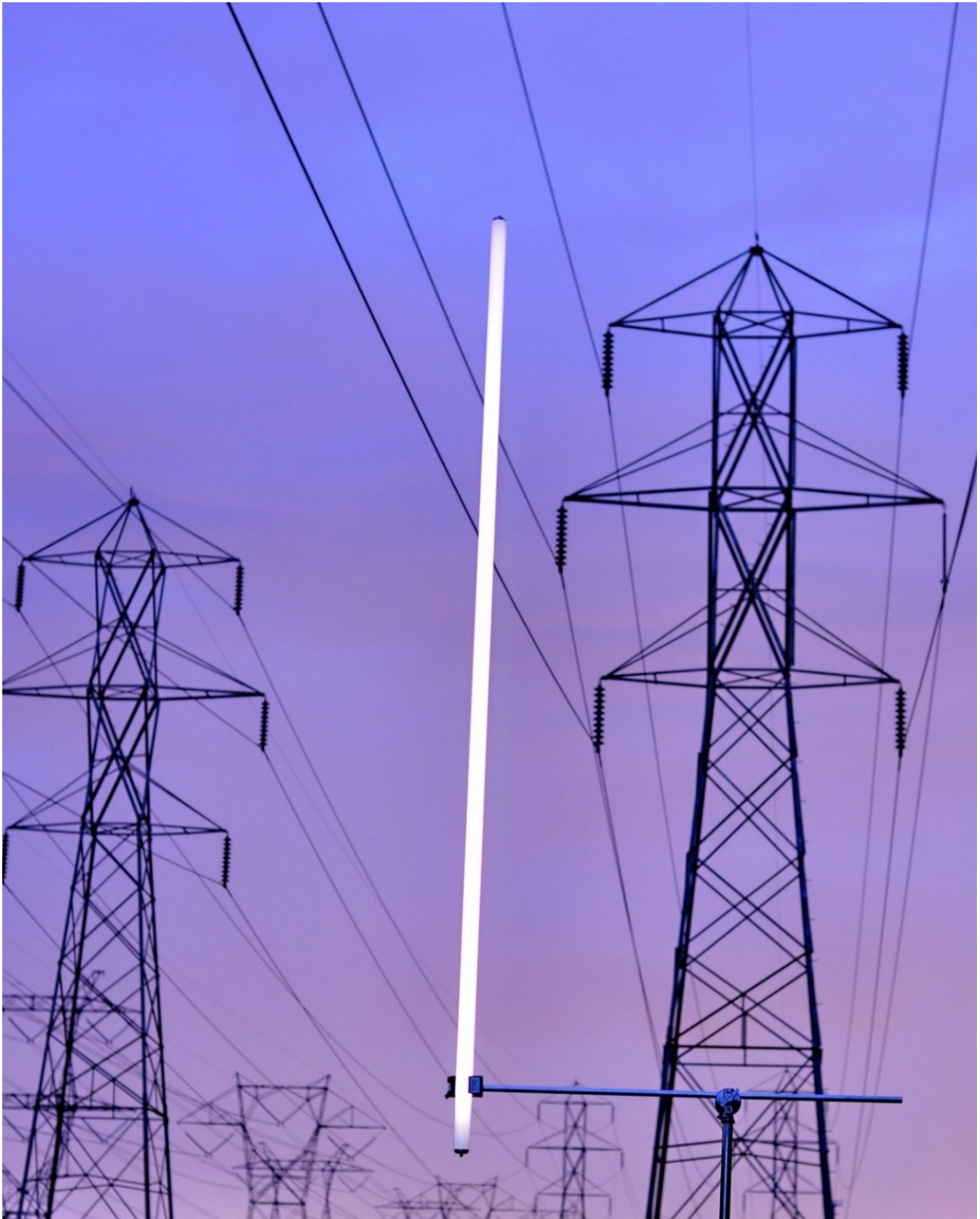
Figure 6.5: A fluorescent tube lit up by electromagnetic fields from a 400 kV powerline. Source: BaronAlaric (2010). Fluorescent tube glowing under electric power lines ( https://commons.wikimedia.org/wiki/File:Fluorescent_tube_under_electric_line.jpg ) CC BY-SA 3.0 creativecommons.org/licenses/by-sa/3.0/ .
