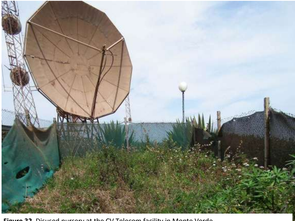
Figure 32. Disused nursery at the CV Telecom facility in Monte Verde.
